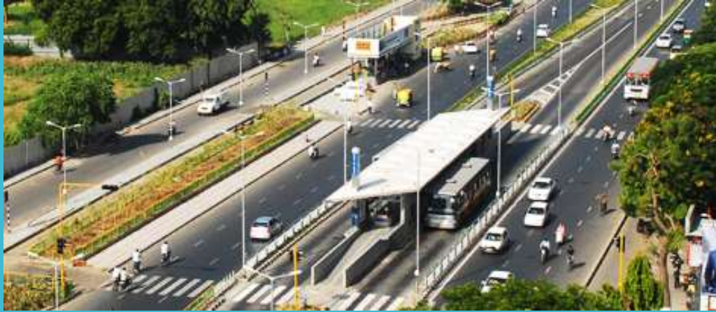
BRTS (Operational – 7 & Under Construction – 5)
