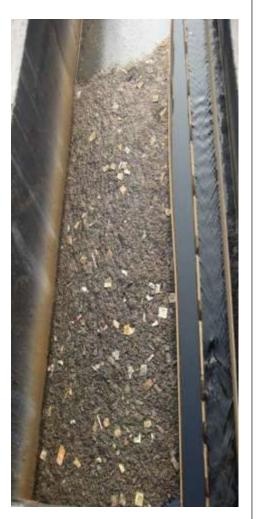
Solid waste - Causing pipe choking and capacity reduction
